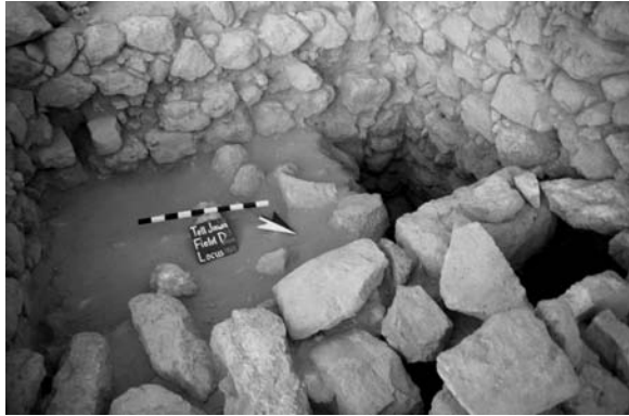
Figure 3.41. Room 609 with Lintel D13:13 in centre right.
